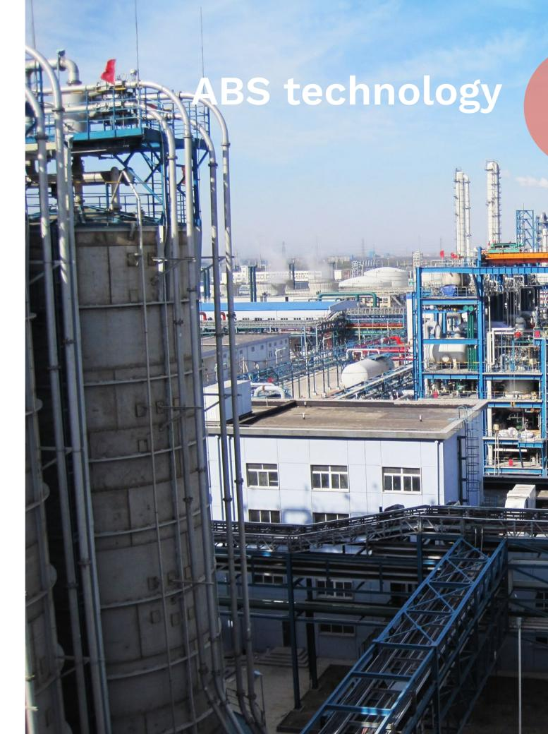
The ABS technology is comprised of four process elements: polybutadiene latex polymerization (PBL), high-rubber graft (HRG) polymerization and isolation, styrene acrylonitrile (SAN) polymerization, and final product compounding. The properties of ABS can be widely varied by using different concentrations of butadiene rubber and acrylonitrile in the copolymer.
