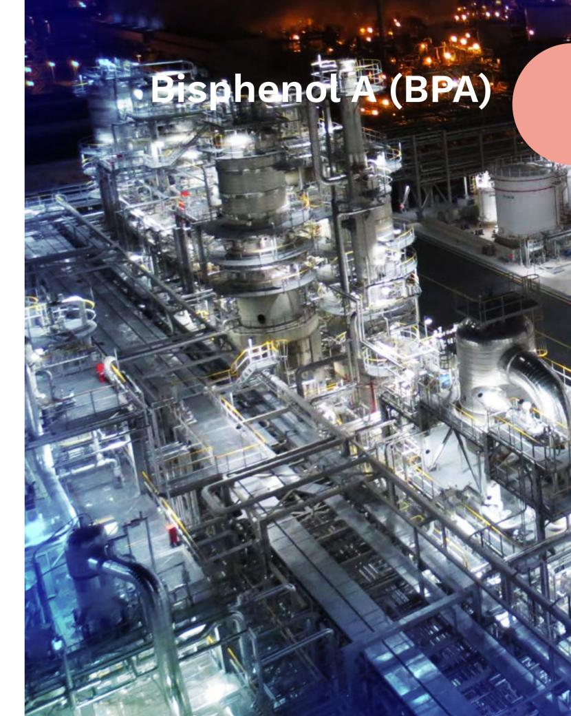
The Badger Bisphenol A (BPA) technology converts commercial grade phenol and acetone into high-purity BPA suitable for polycarbonate, epoxy resin, and other chemical applications.
