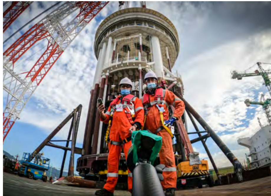
Cybernetix team on Coral FLNG construction yard
