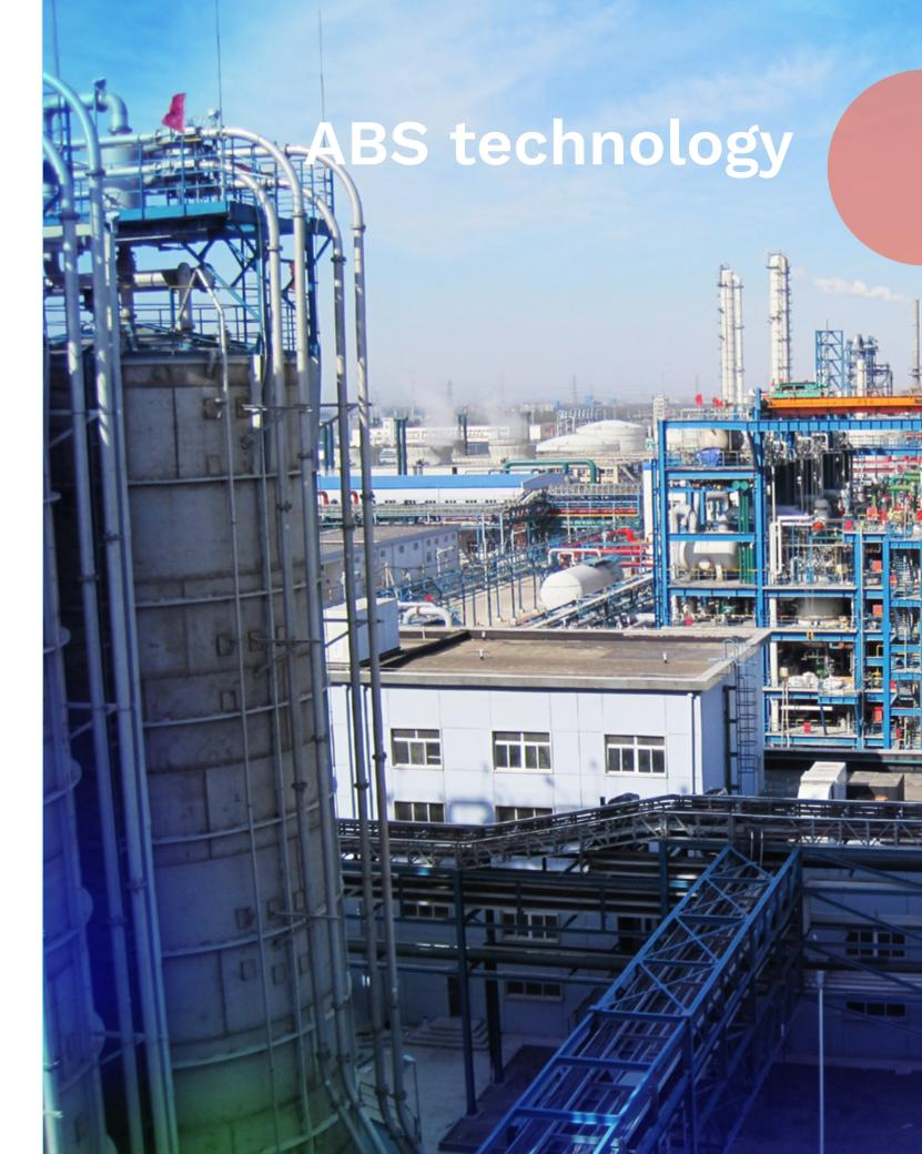
The ABS technology is comprised of four process elements: polybutadiene latex polymerization (PBL), high-rubber graft (HRG) polymerization and isolation, styrene acrylonitrile (SAN) polymerization, and final product compounding. The properties of ABS can be widely varied by using different concentrations of butadiene rubber and acrylonitrile in the copolymer.
